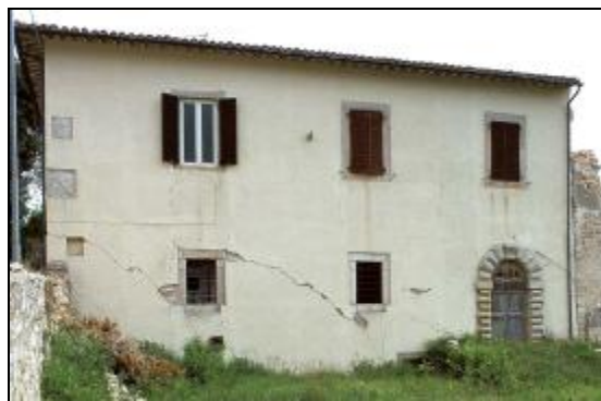
Slika 13. Umbrija, 1998: kose pukotine u zidovima zgrade od kamena Figure 13. Umbrija, 1998: diagonal cracks in the stone walls of a building
