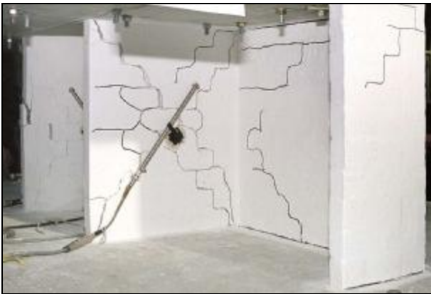
Slika 7. Oštećenja 3. stepena kod graničnog stanja maksimalne otpornosti (Model M1-1c, \Phi=0,9\% ) Figure 7. Grade 3 damages with the limitation state of the maximum resistance (Model M1-1c, \Phi=0.9\% )
